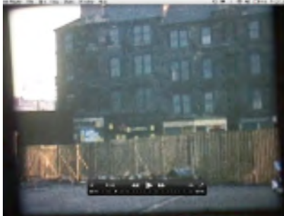
Figure 1. 542 St Georges Road Glasgow, circa 1967 immediately prior to demolition
